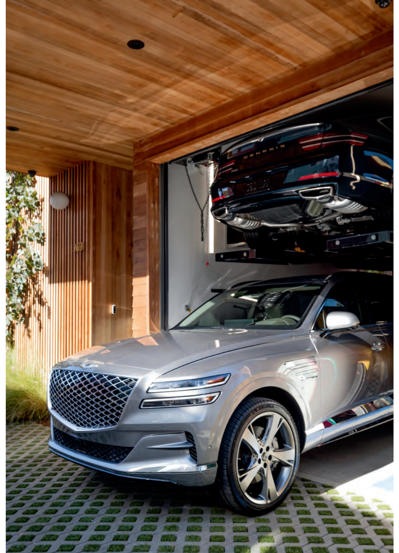
A hydraulic lift accommodates two cars in this single-wide and double-deep garage.
